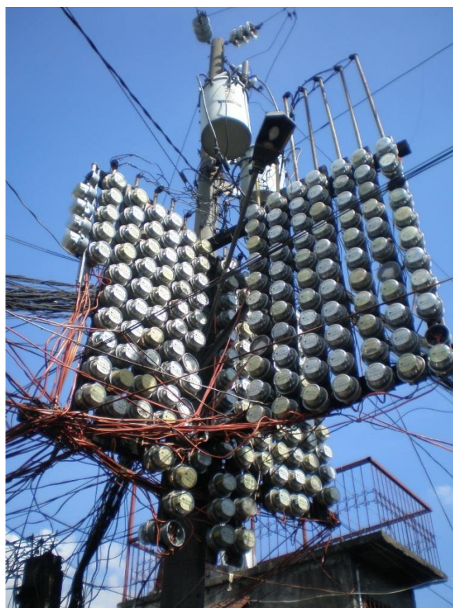
FIGURE 15 METERS AND SUBMETERS IN AN INFORMAL SETTLEMENT (PHOTO BY AUTHOR)
